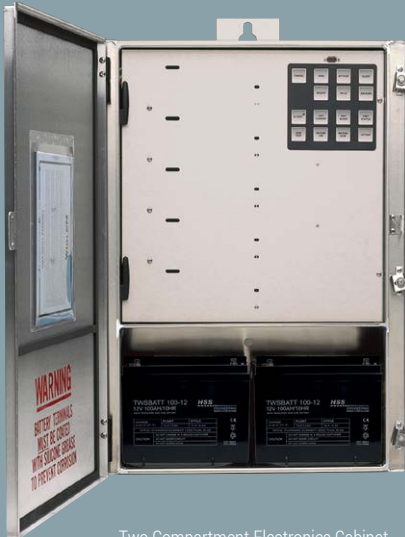
Two Compartment Electronics Cabinet
