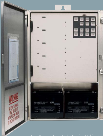
Two Compartment Electronics Cabinet
