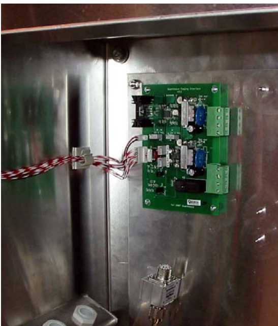
Fig. 3 Paging interface installed in a TWS series cabinet.
