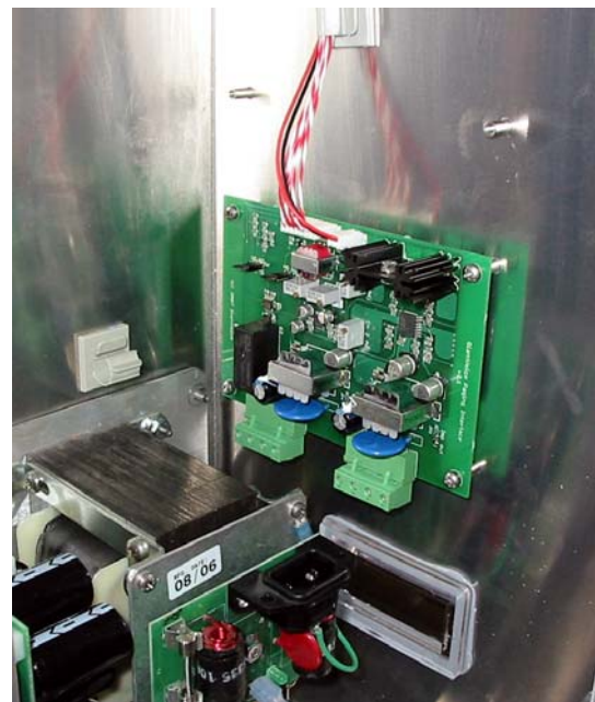
Fig. 4 Paging interface installed in a WPS series cabinet.
